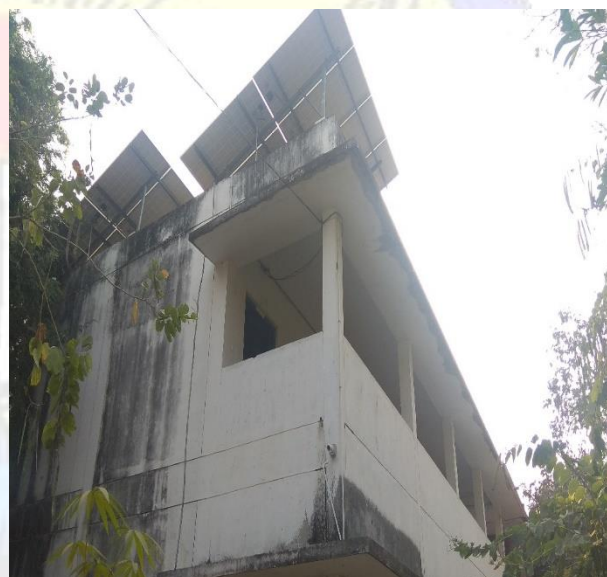
Figure 1: Solar PV panels at Roof of the Building
